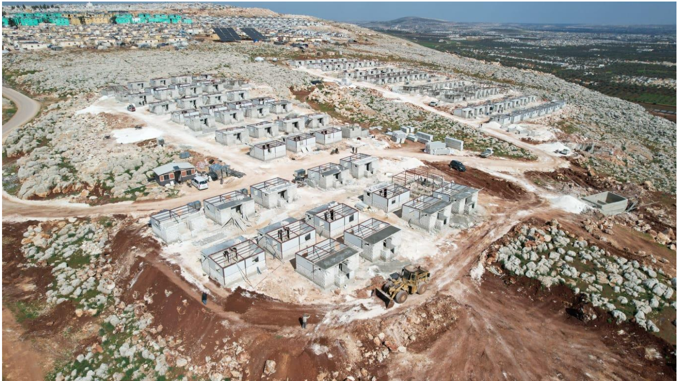
With support from the people of Taiwan, dignified shelter units were installed for earthquake-affected households.
